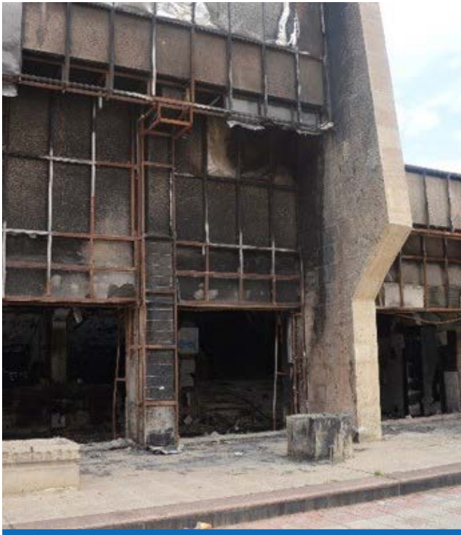
The exterior of University Hall, before FFS rehabilitation.
