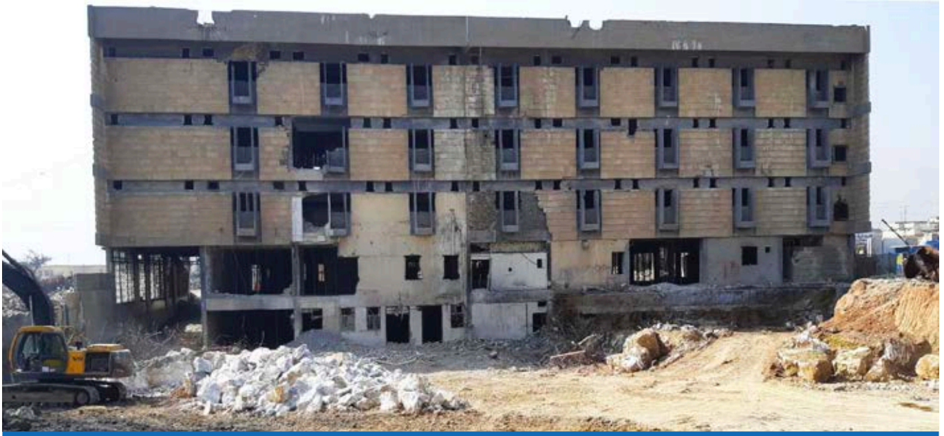
Rehabilitation of Al-Batool Maternity Hospital started in Q1.
