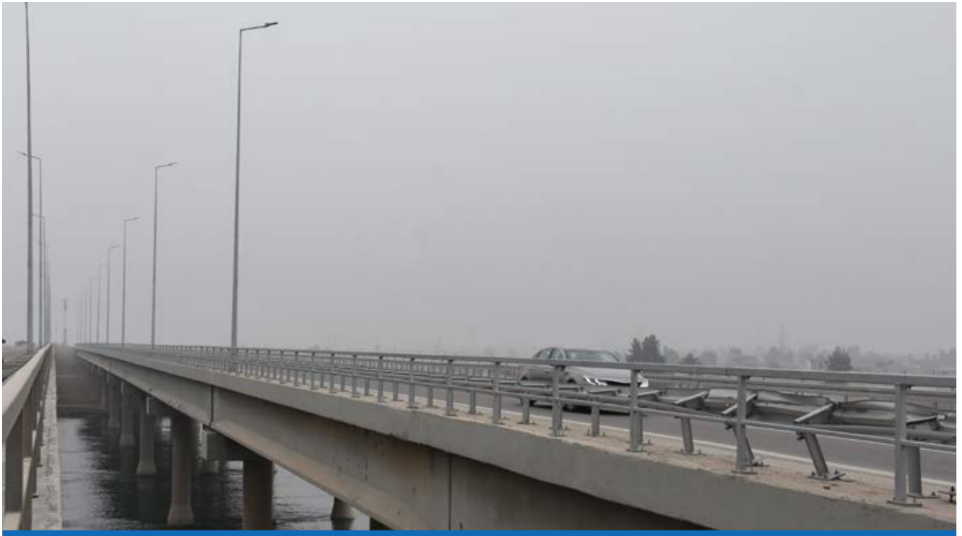
The rehabilitation of the Palestine Concrete Bridge was completed
