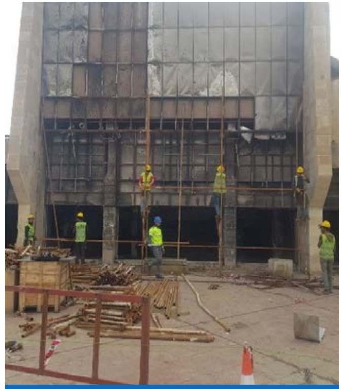
Work is progressing on the exterior of the University Hall
